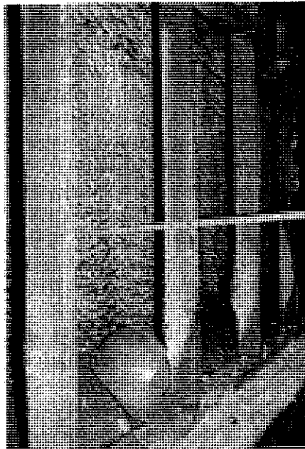
A view of combustible concealed space between the wood-framed interior surface and the plastic foam insulation.
