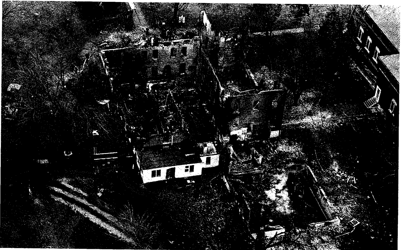
Katie Jane Nursing Home, Warrenton, Mo. Remains of Annex in right foreground.
