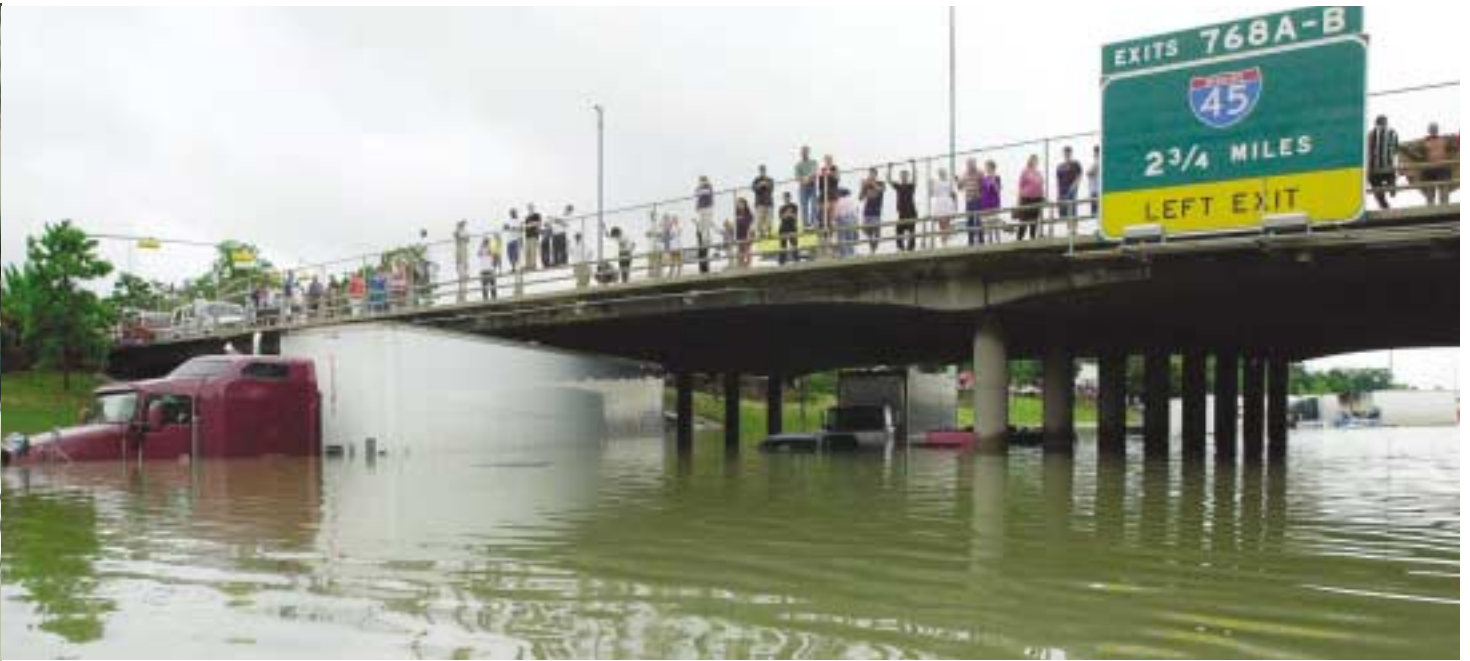
Onlookers stand on an overpass where flood waters covered Interstate 10 in Houston, on June 9, 2001, as Tropical storm Allison swamped Southeast Texas.
