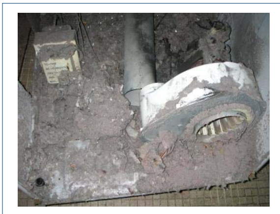
Disconnected vent pipe & lint accumulation inside dryer. Photo provided by J. Doran, NSC Marine Section WTG.
