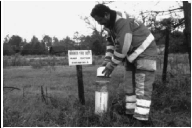
Figure B.5.6(a) A dry hydrant innovation has eliminated the top 90-degree or 45-degree elbow on each hydrant. (Photo by Nahunta Volunteer Fire Department, NC)
