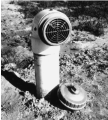
Figure B.5.1(a) Dry hydrant.
