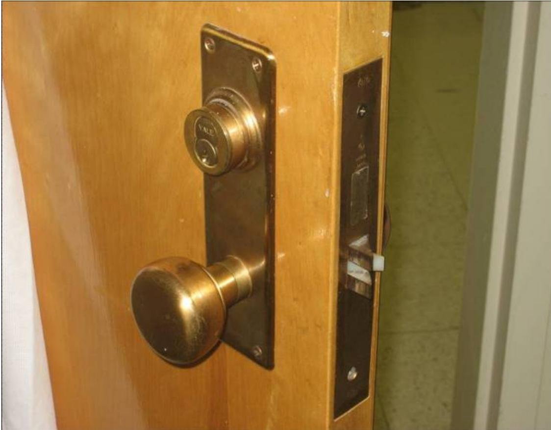
**Figure 2. Door Requiring Two Operations**
