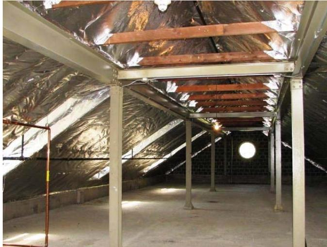
**Figure 1. Unprotected Steel (ref: 19.1.6.5)**
