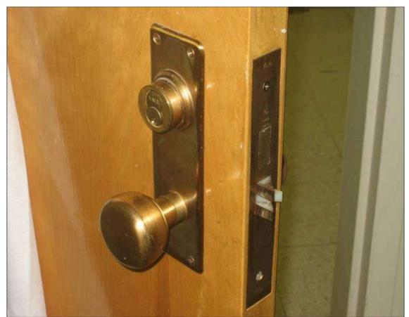
Figure 1. Door Requiring Two Operations
