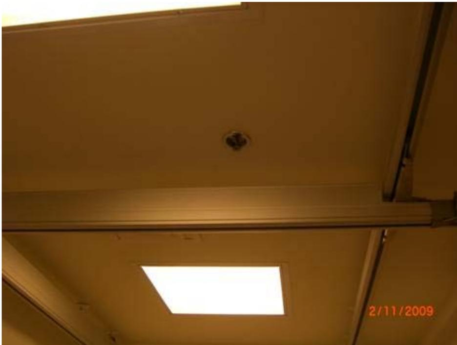
The spacing of the sprinkler relative to the two fixed rails are installed to meet all the obstruction rules of NFPA 13. The moving rail, perpendicular to the fixed rails, will move and can obstruct the sprinkler during its movement when it is located near the sprinkler and it can obstruct the sprinkler if it is "parked" near the sprinkler.
