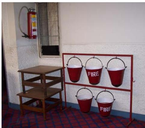
*Photo of fire protection devices in a hotel in India. An ABC fire extinguisher, tables for people to climb out and 5 buckets ,2 with water and 3 with sand.*
