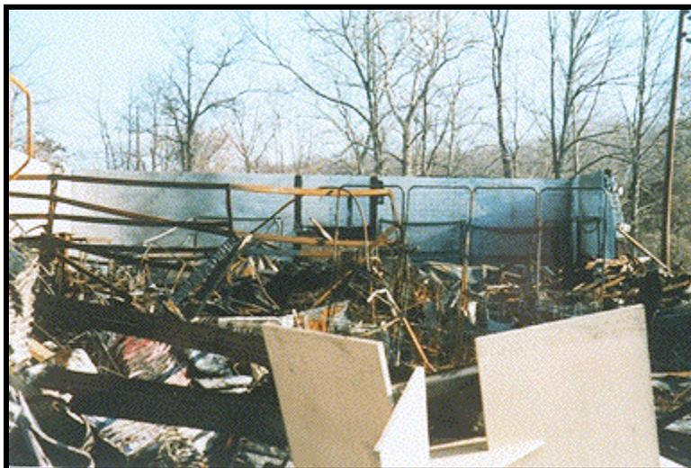
The building was 60 ft (18.3 m) wide and 120 ft (36.5 m) long. It had wood-frame exterior bearing walls in one section and masonry block exterior bearing walls in all other areas. Lightweight wood trusses carried the store's roof over a clear span of 60 ft (18.3 m). The building did not have any fire detection or suppression systems.
