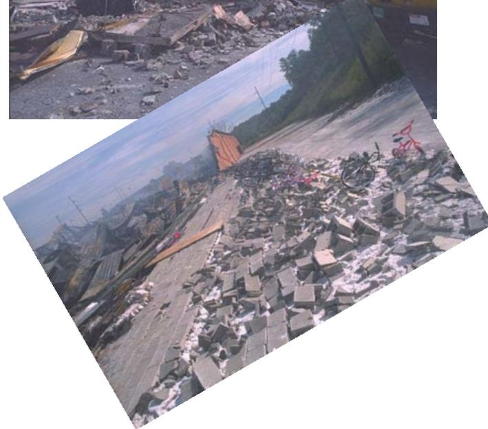
A fire in a sprinklered retail store highlighted the hazardous associated with the improper storage of LP cylinders within the building. A leak from one of the cylinders created a gas cloud that was then ignited, seriously damaging the buildings sprinkler system. The ensuing fire and additional explosions totally destroyed the store and its contents.
