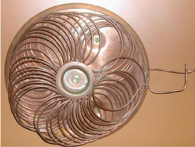
“Typical” pneumatic heat detector
