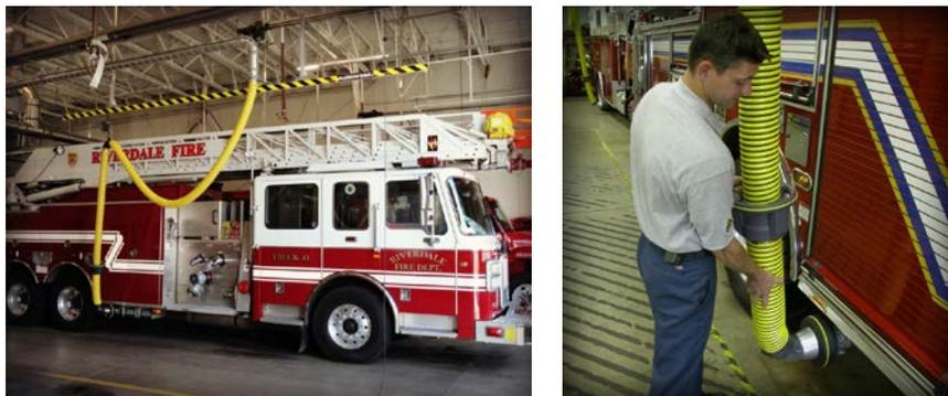
Figure 4: Local Tailpipe Exhaust System Example
