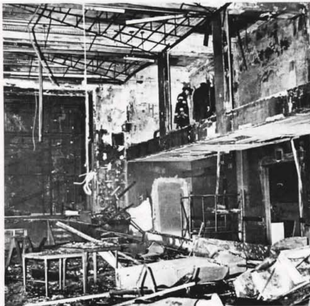
This general view of the auditorium shows the remains of the lumber and other building materials that were in the auditorium. The fire is thought to have been set at the end of the balcony to the right of the stage, where the firemen are standing.
