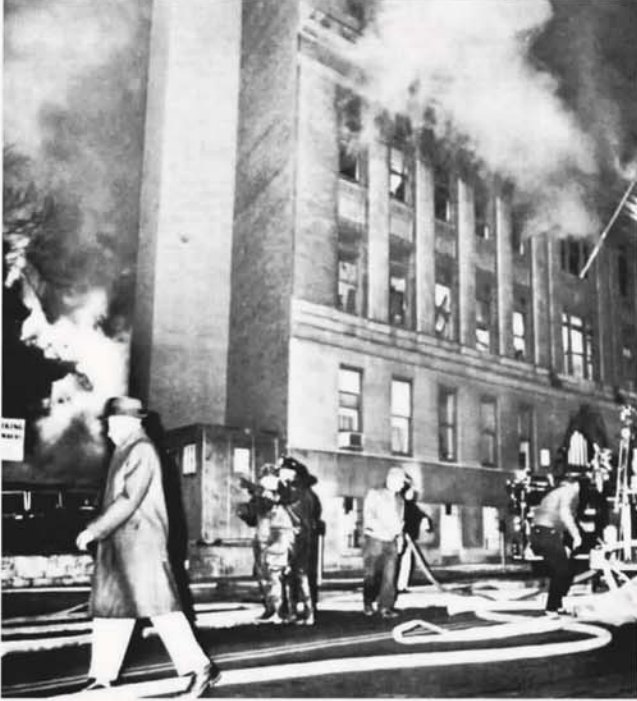
This photo was taken looking toward the northwest corner of the building. The tall narrow structure on the left is the new elevator shaft added as a part of the extensive remodeling program that was going on at the time of the fire. Although the flames at the left seem to be coming out of the lower story of the building, they are actually coming from the second- and third-story windows of the auditorium and balcony. WIDE WORLD
