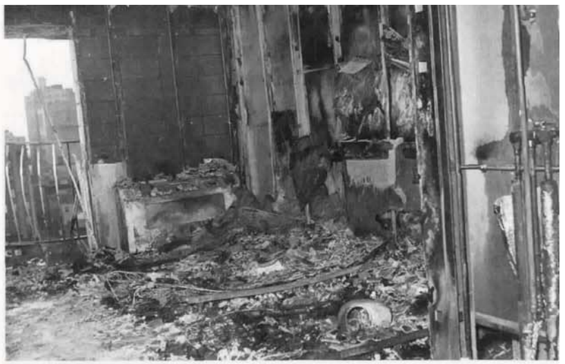
Each room has an air conditioner built into the masonry-block wall, as shown here. The doorway to the railed-in balcony is at the left.
