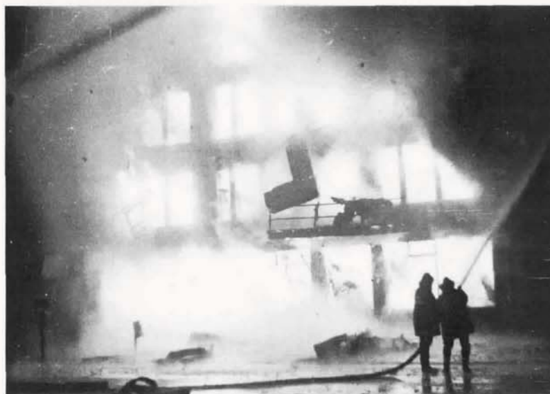
Soon after fire fighters arrived they had to face the conditions shown above. The heavy fire prevented any attempts to enter the building or effect rescue.
