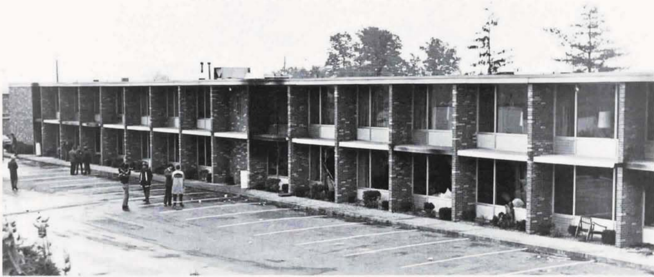
The fire originated in the first-floor room to the right of the white barrel in the center of the photo. Flames exposed the balcony of the room directly above.
