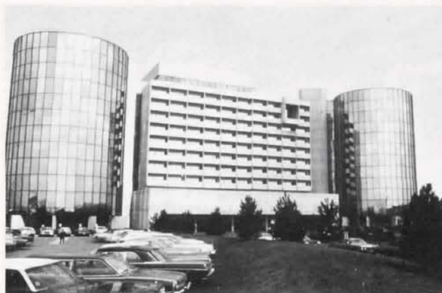
The atrium is within the center balconied building. Two of the four towers are at left and right. NFPA
