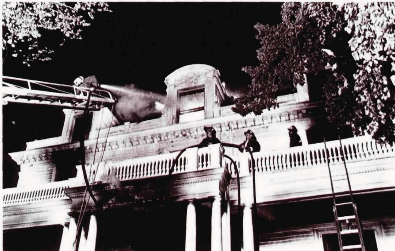
Photo 1. A substandard heating system installation, nonfirestopped concealed spaces, open stairways, and lack of automatic fire protection combined to cause this fatal fire. UPI
