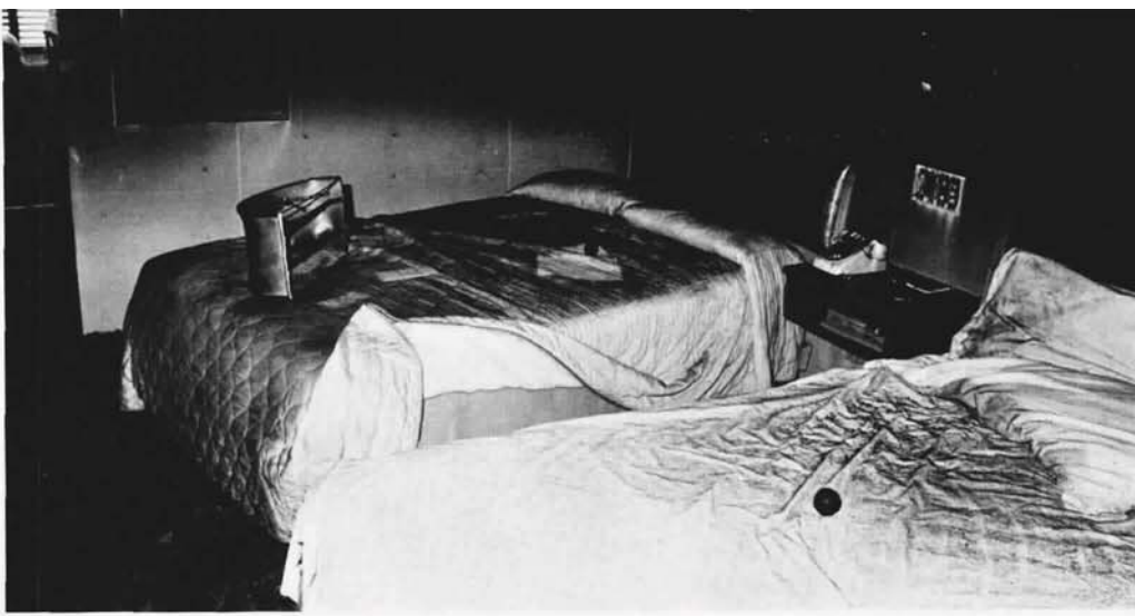
Smoke damage to room resulting from TV set fire.
