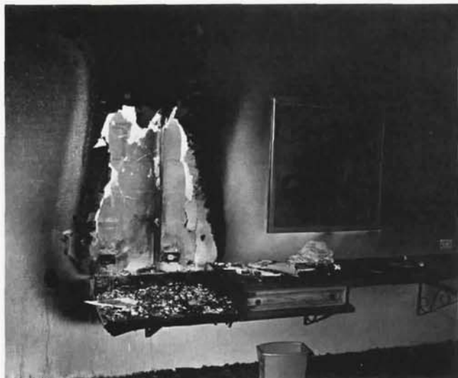
Photo 1. Damage to wall covering directly over TV set location.
