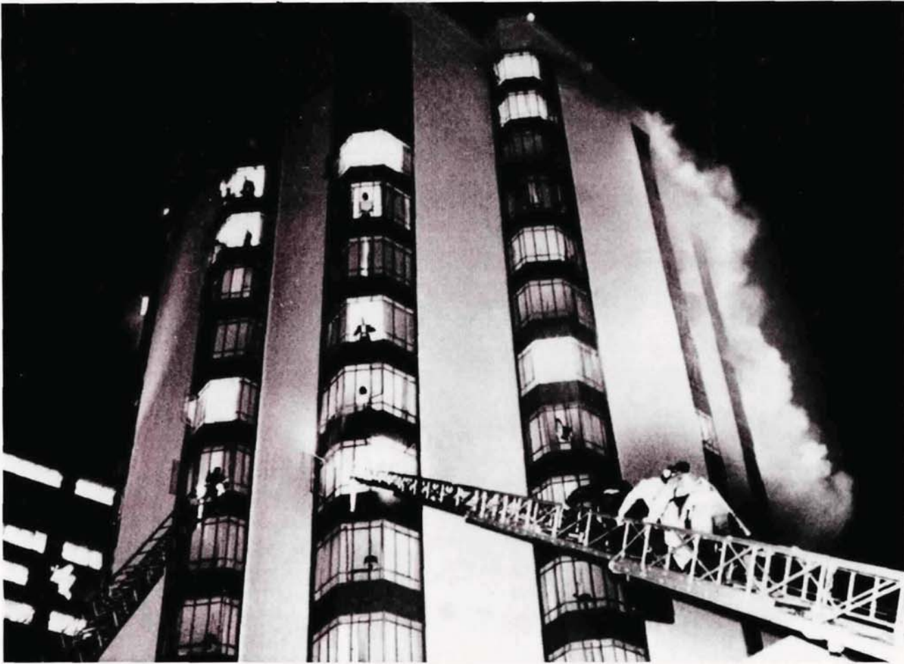
Guests on the upper floors of the 15-story University Tower Hotel had to "sit it out" as a fire on the mezzanine floor filled corridors and a stairway with smoke. The Fire Department's 100-foot aerial ladders could not reach above the eighth floor.
