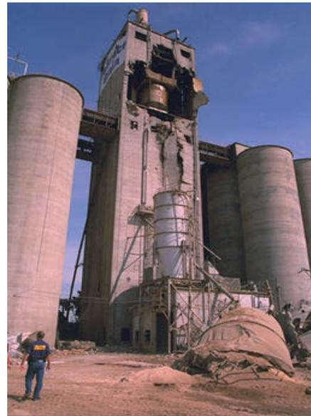
***Figure 1: Photo showing damage to headhouse structure (NFPA)***
