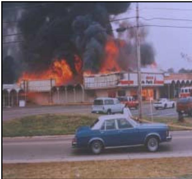
exterior bearing walls were constructed with unprotected steel frames and two were constructed with masonry block. Lightweight wood trusses with a clear span of 50 ft (15.2 m) supported the store's roof. Because the facility was an auto parts store, it contained a wide variety of combustible and noncombustible materials, flammable auto paints (liquid and aerosol), and other flammable and combustible liquids. Most packaging materials and some shelving materials were also combustible.
