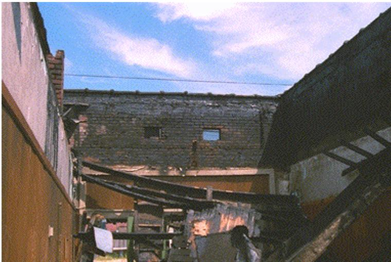
**Photo No. 6: View showing attic space at front (north) of restaurant. The blackened bricks indicate the attic area (NFPA)**
