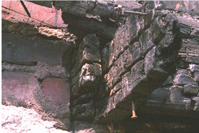
**Photo No. 1: Roof joist ends at brick wall in florist shop (NFPA)**
