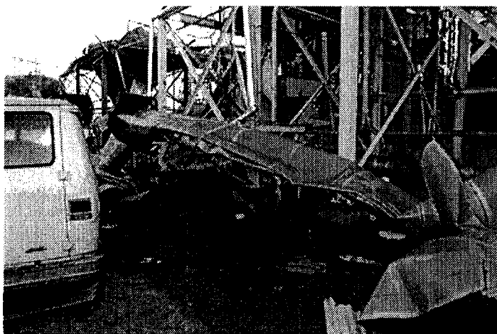
Picture of the damage to some of the ductwork on the south-east side of the building.
