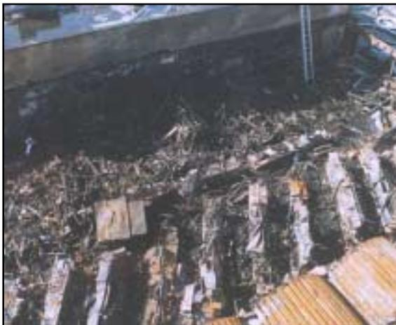
The fire occurred when a utility worker damaged the electrical service drop conductors on the outside of the store. Electrical arcing inside the store ignited fires that quickly involved the wood trusses supporting the roof and ignited a fire in the area of an electric hot water heater. Though some of the fire was visible to anyone in the occupied area of the building, much of the fire was hidden in the concealed space above the store's ceiling, and the fire was able to
