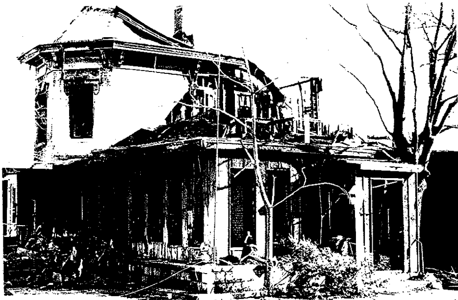
Photo 1: Northwest corner of the building showing the one story addition. The point of origin was a sofa located in the apartment in this corner of the building.
