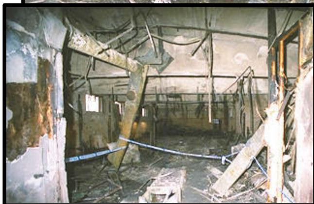
**Factors contributing to the loss of life in this incident include the overcrowded conditions in the hall, combustible storage in a stairwell and the lack of a fire alarm system in the building.**
