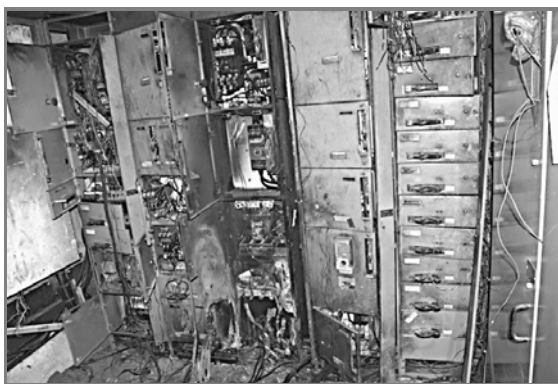
Figure L.9(b) Close-up View of Main Circuit Breaker Lug Failure.
