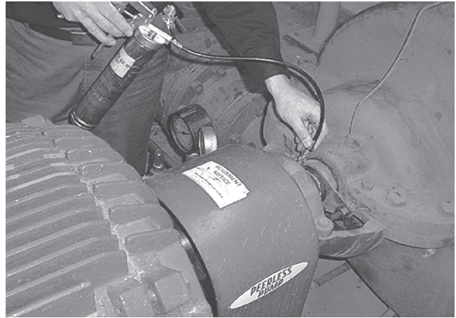
EXHIBIT 4.3 Pump Shaft Bearing Lubrication
